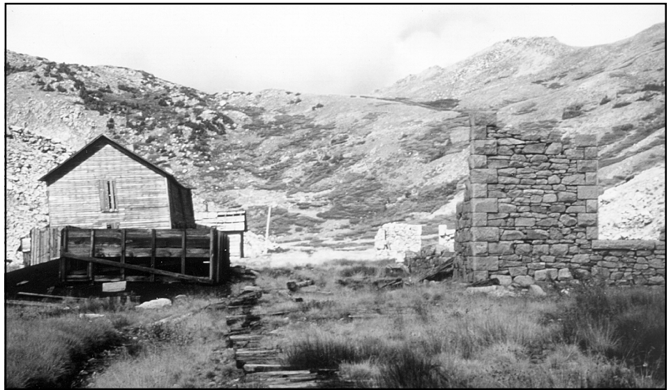
The boarding house and what remained of the engine house on October 2, 1948. It was still possible to roam around inside that old building and wonder just what it must have been like when in use. There surely must have been some animated talks.
